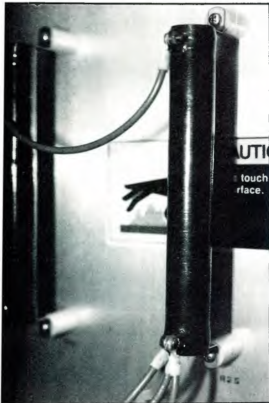
Check resistors, particularly high-power units, regularly for signs of premature wear because of excessive heating.
